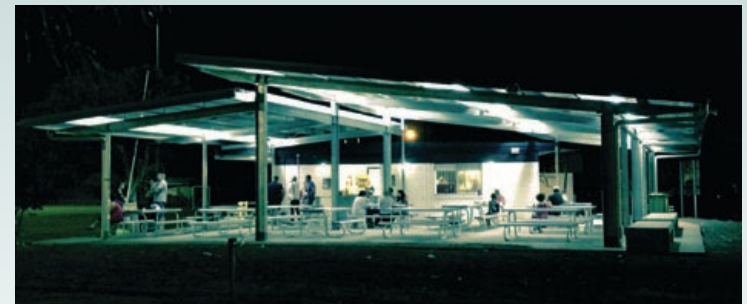
The final stage of the clubhouse expansion for Brothers Junior Rugby Club was the newly completed undercover area.
